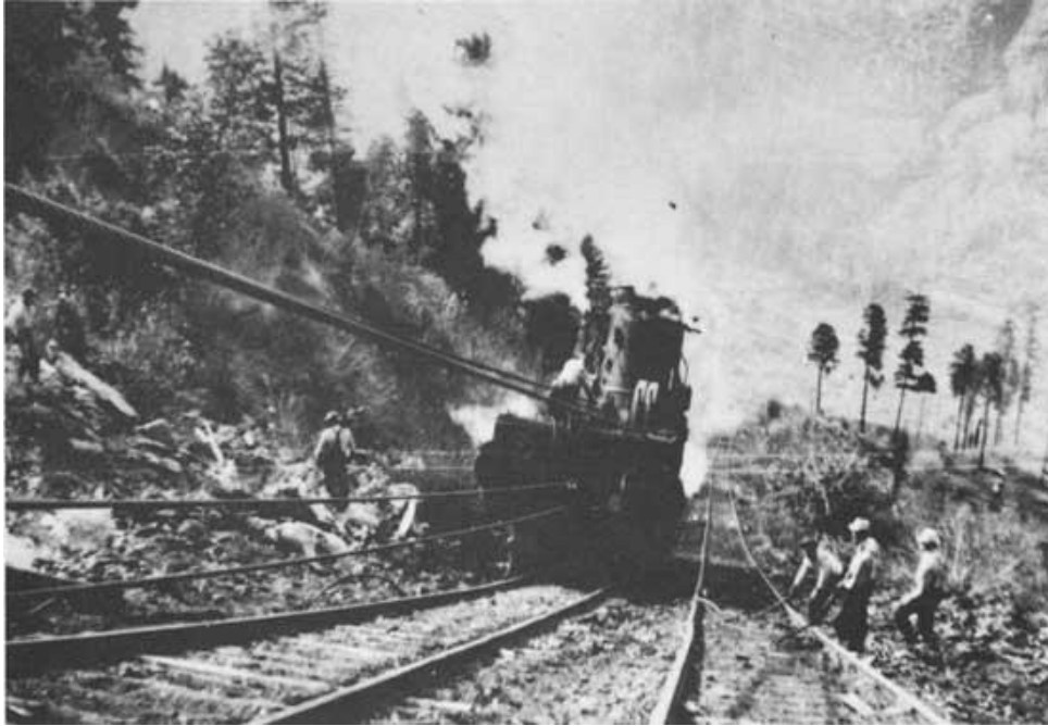
Moving a donkey on incline rails in the North Fork Willamette sale area, 1930.
