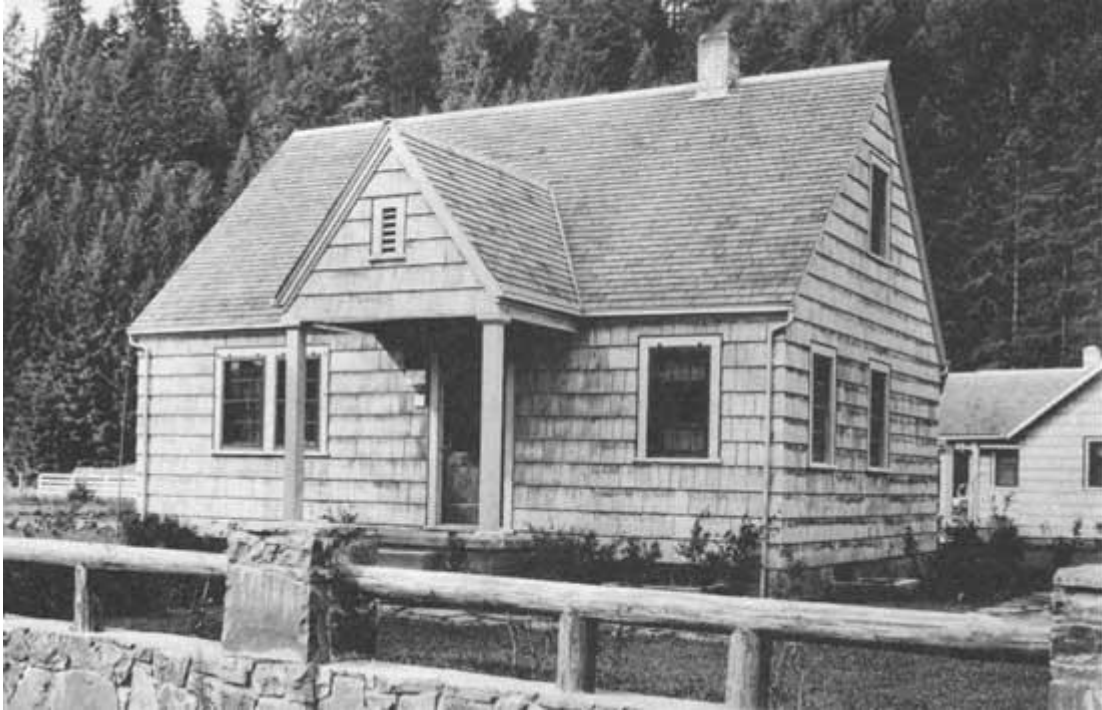
West Boundary Ranger Station, 1936.
