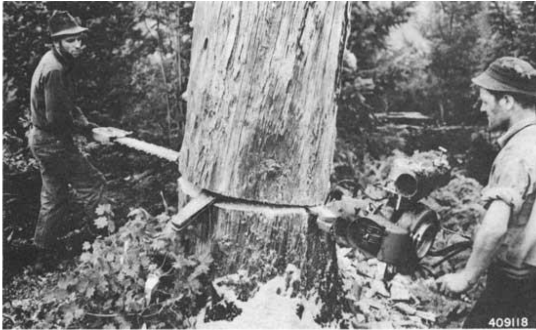
Snag falling with a gasoline driven power saw on the Tumble Creek Fire near Detroit, 1941.
