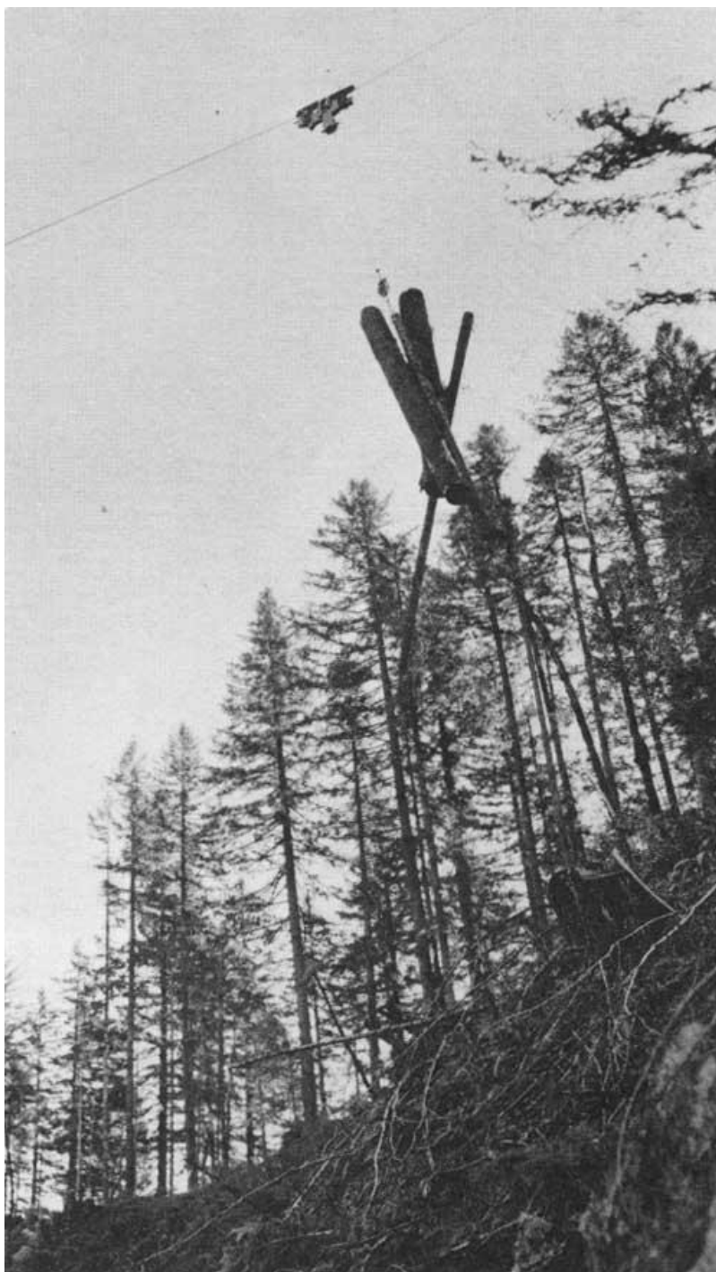
Wyssen Skyline Crane - logs being lifted to the carriage in the H.J. Andrews Experimental Forest, c. 1970.
