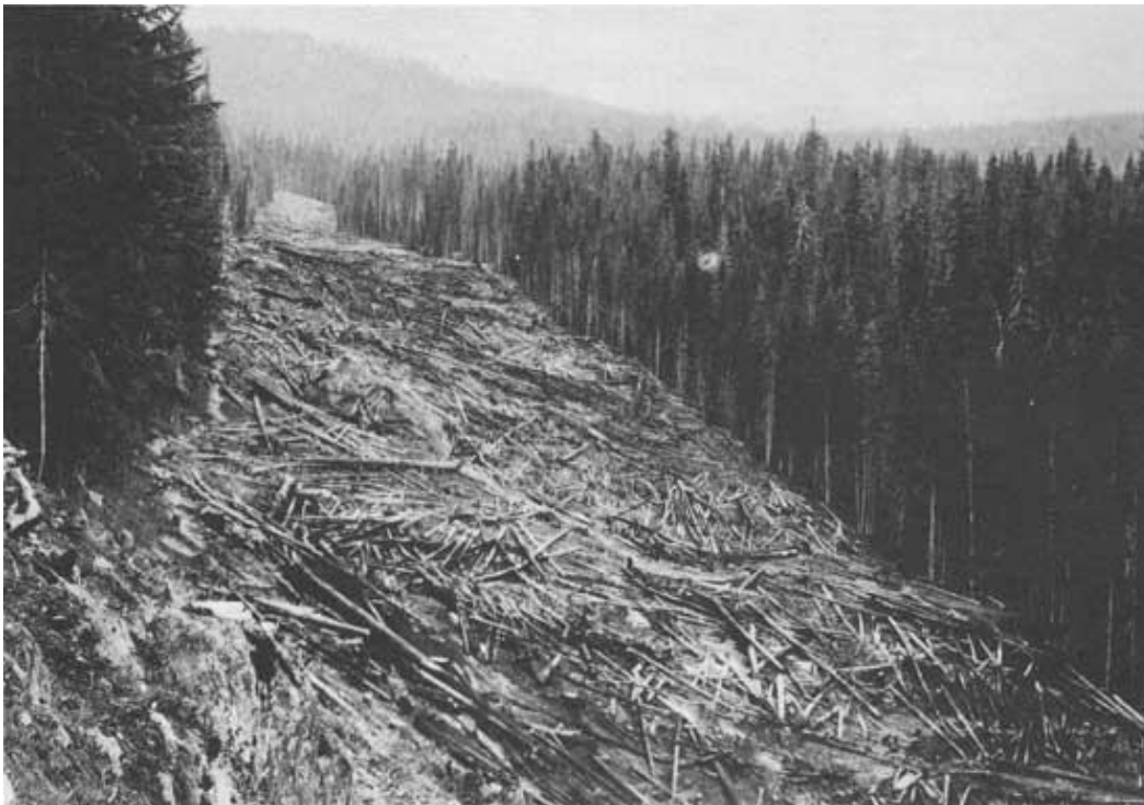
Clearing the railroad right-of-way near the summit of the Cascade Range. Natron cut-off, Southern Pacific RR, 1925.
