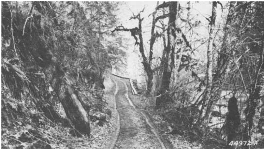
McKenzie River Highway above Blue River (note the log guard rails), 1920.
