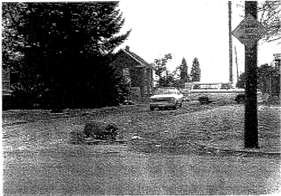
Fig. 76 Unpaved Streets: 24th & Wygant (T. Ward)
