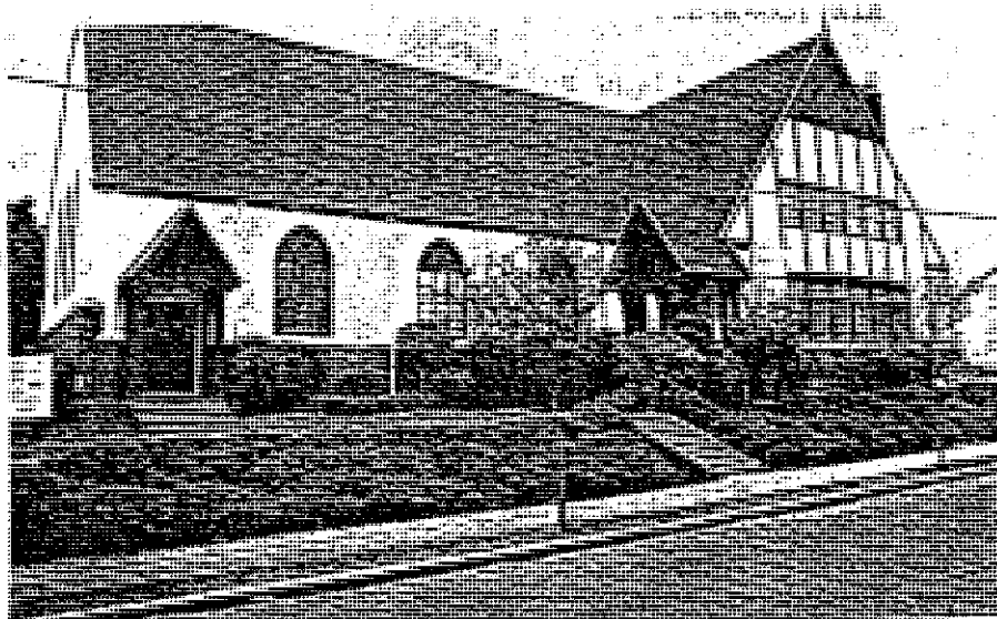
4635 NE 9th Avenue. Highland Congregational Church, 1926.
