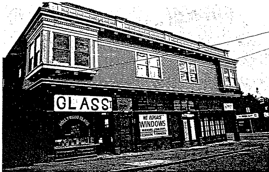
2926 NE Killingsworth Street. Streetcar Era Commercial Apartment House, 1911.
