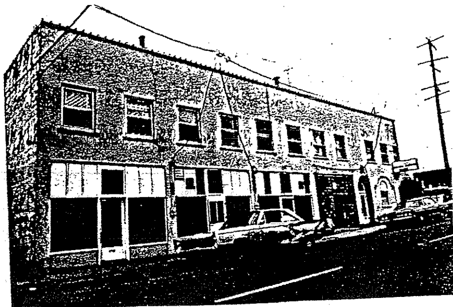
3000 NE Alberta Street. Alberta Theatre, 1926.
