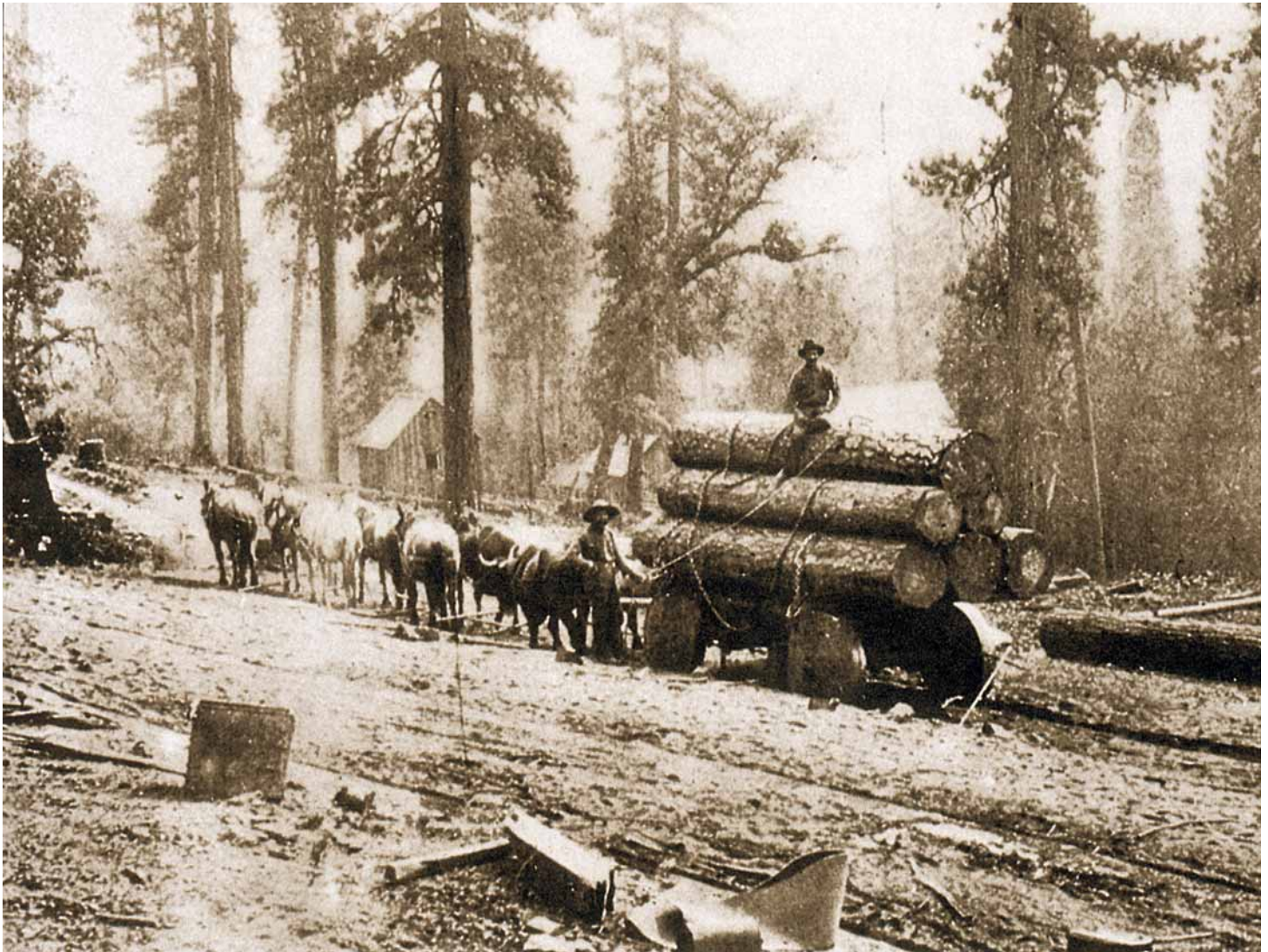
The caption for this photograph from the 1900 USGS report reads, "Common method of hauling yellow-pine logs to sawmill." Compare the size of these logs with the log and loggers shown in the nearby 1922 postcard. Early sawmill records indicate logs of the size shown on the postcard were the exception rather than the rule. Most of the earliest logs were turned into railroad ties, mine timbers, firewood and bridge pilings, products best made from smaller trees. Besides, the equipment needed to transport the largest logs to mills did not yet exist, and they were frequently burned as fuel in "steam donkeys," steam powered machines used to drag logs from hillsides to railside.
