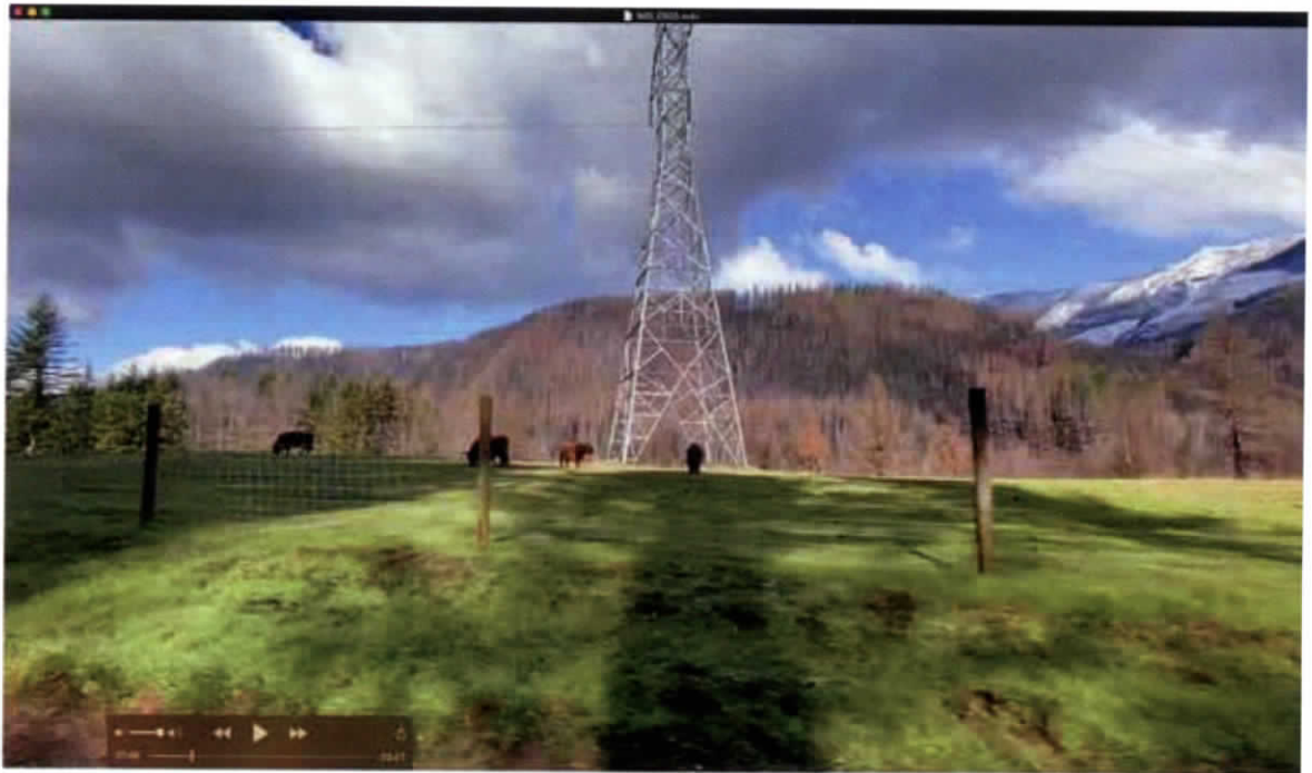
Fig. 1, Powerline right-of-way and grazing cattle. Beachie Creek Fire aftermath. November 8, 2020 video-clip by McKenzie Peters, NW Maps Co.
