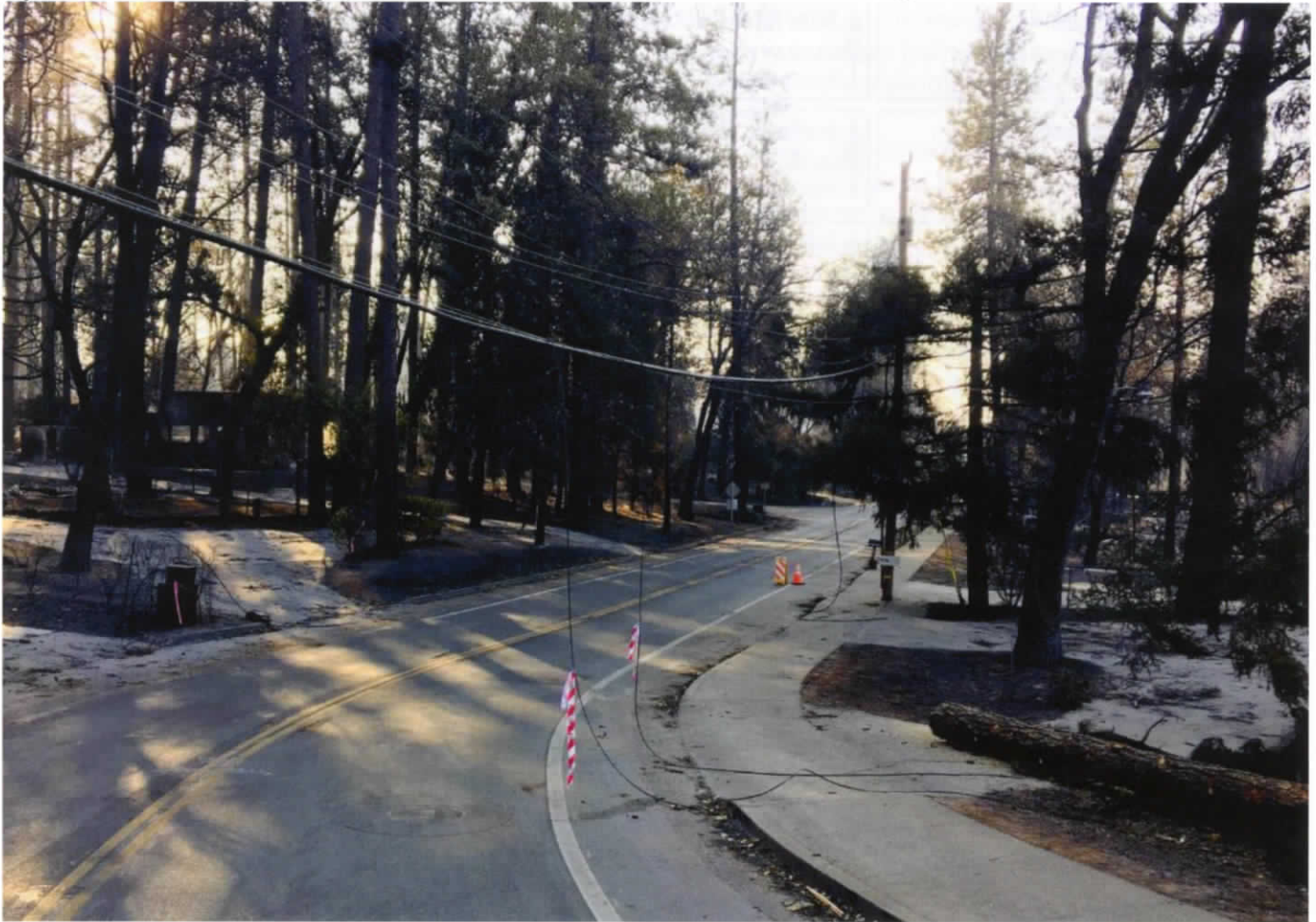
Inciweb (USFS) photo of downed powerlines on November 18, 2018 in Paradise.
